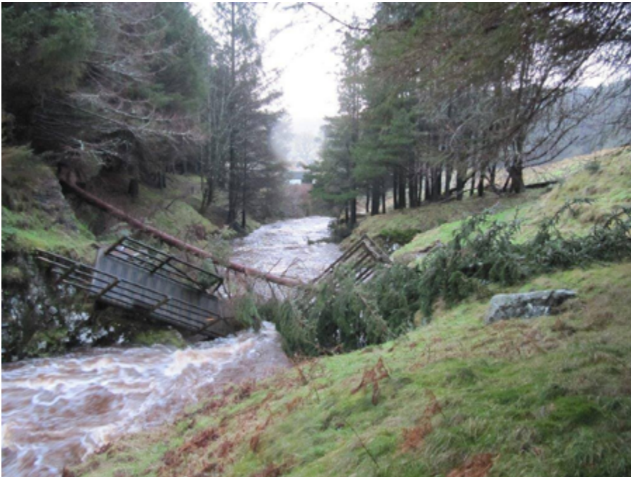
Access interrupted due to a damaged bridge in the Northumberland National Park
